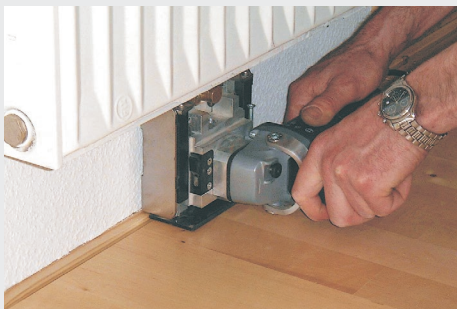
Cutting expansion joints under radiators
